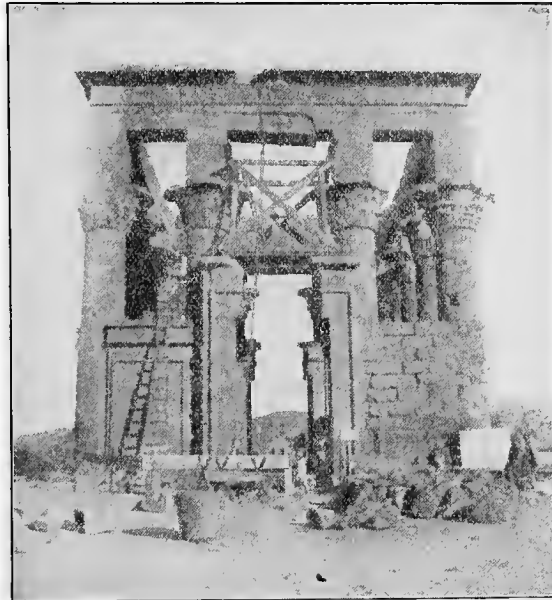
THE KIOSK AT PHILÆ IN PROCESS OF UNDERPINNING AND RESTORATION, JANUARY, 1902.
